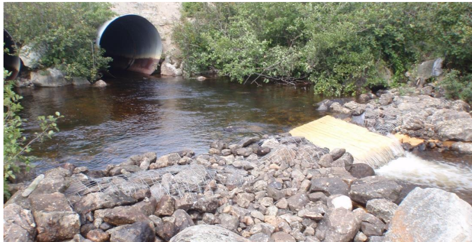
Figure 1: Low head weir located downstream of Highway 320.
